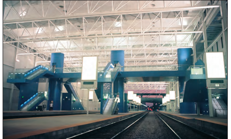
The mezzanine, spanning all five tracks, allows passengers to walk above the tracks to reach the three boarding platforms.
