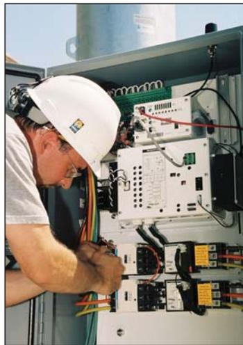
*Roman electrician Mike Gerhardt connects the lighting control cabinet to one of the four 100 ft. tall lighting poles after it had been precisely aligned to match the engineered lighting coordinates.*
