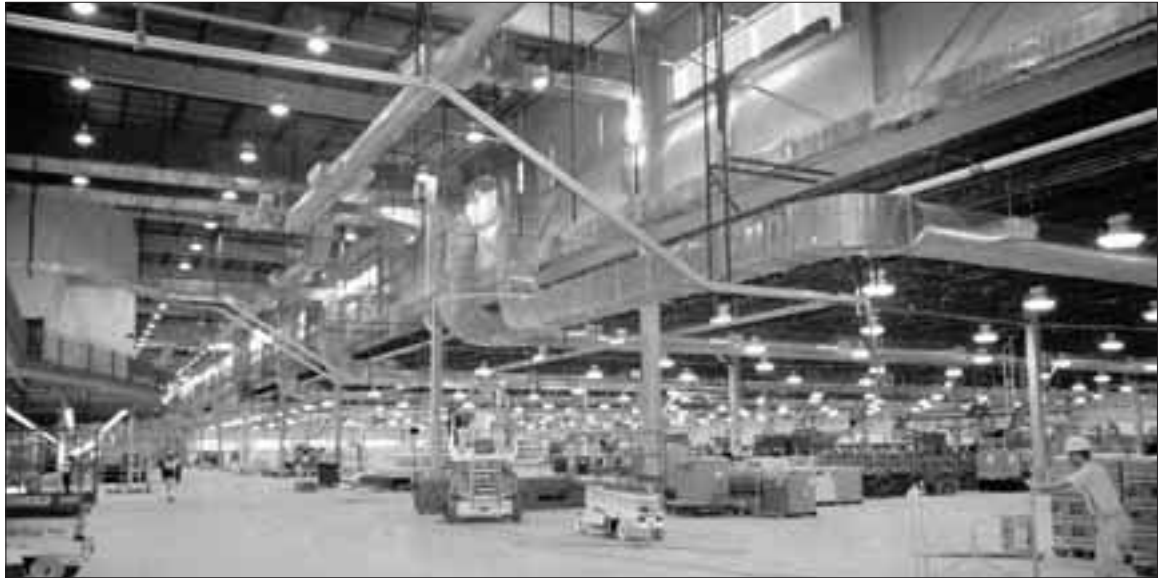
The well-lit new Journal Sentinel newspaper production plant is illuminated by 4,650 fluorescent and HID lamps installed by Roman Electric crews.
