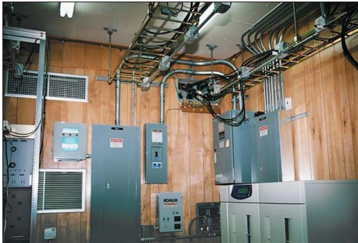
*Instantaneous backup power is provided by UPS equipment like this three phase battery powered system.*
