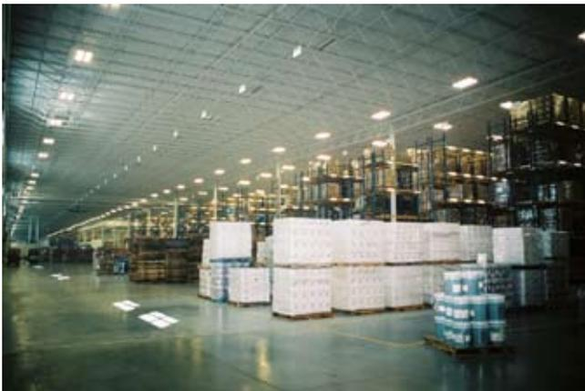
*The well-designed lighting system in JohnsonDiversey's LEED certified 550,000 sq. ft. distribution center is expected to reduce energy usage by 60% and save up to \$90,000 per year. The warehouse is lighted by high-output T5 high-bay fluorescents with occupancy sensors and lighting controls.*
