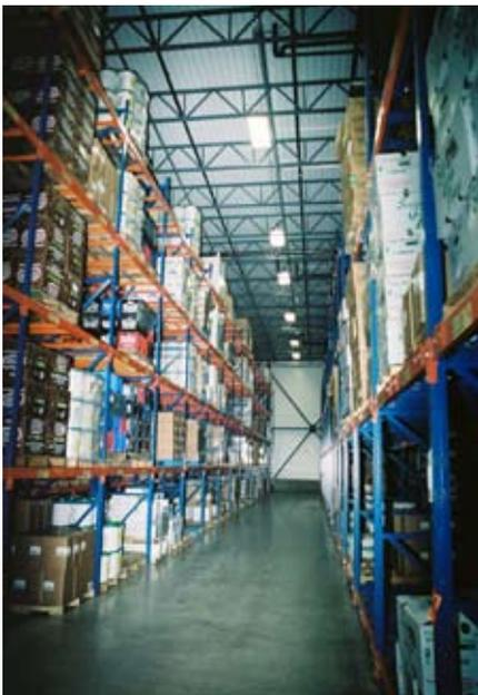
*Dierks Waukesha Foods achieved substantial lighting savings by having Roman Electric replace older high pressure sodium and metal halide lamps with energy-efficient high bay fluorescents. With the new lamps, occupancy sensors that only turn lights on when someone enters the aisle, Focus On Energy rebates and federal tax deductions, the food distribution company is saving at least \$5,000 per month.*
