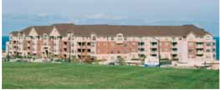
Roman was the electrical contractor on The Landing at Park Shore. The 301-unit complex, possibly the largest condominium complex in Wisconsin, offers spectacular views of Lake Michigan.
