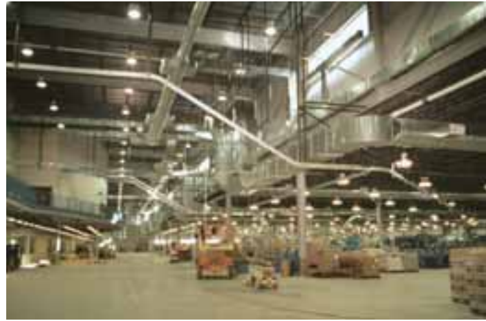
Above: The well-lighted new Journal Sentinel newspaper production plant is illuminated by 4,650 fluorescent and HID lamps installed by Roman Electric crews.
