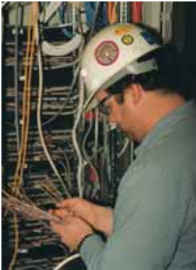
Roman TechNet foreman Dan Patterson installs fiber optic and copper voice and data cable in Nitto America's new 180,000 sq. ft. facility in Pleasant Prairie. Roman was design/build electrical contractor on the huge project.
