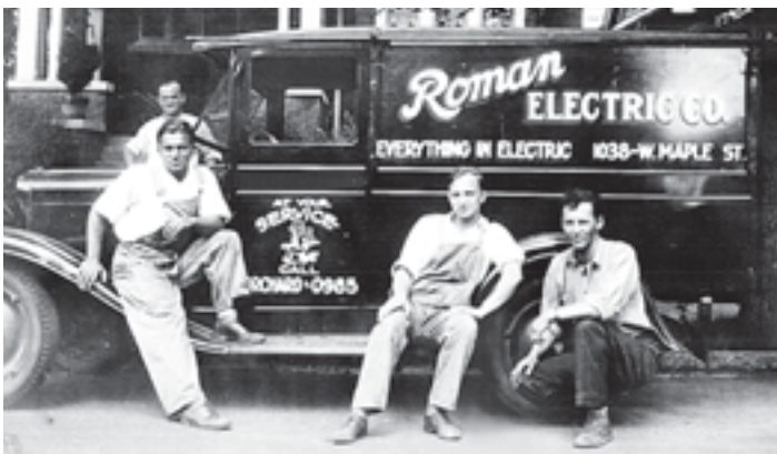
Roman Rose (second from right) poses with his complete electrical crew and their first new service truck in 1933.
