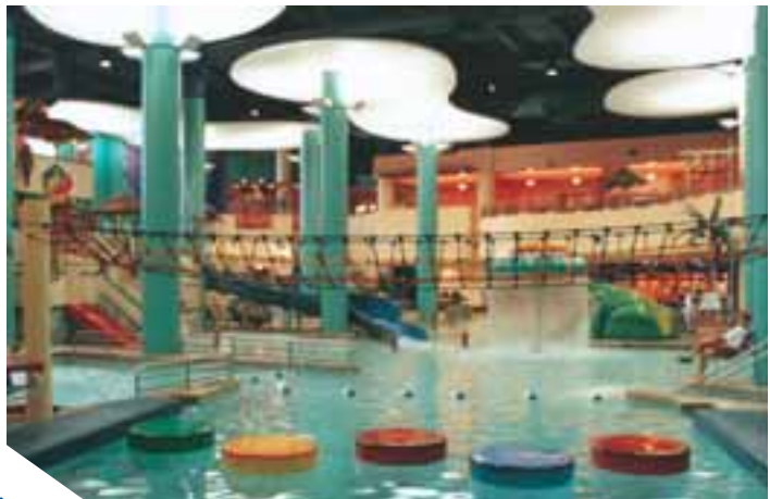
A three-story, 20,000 sq. ft. water park was part of the $40 million expansion of the Hilton Milwaukee City Center. Roman, heavily involved in the renovation, installed power and lighting in the water park.
