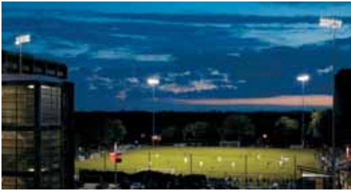
For the first time since the UWM Panther's soccer team began playing its home games on campus at Engelman Field in 1973, it can now play attendance-boosting night games. Roman Electric installed a new state-of-the-art field lighting system with four 100 ft. tall prewired light poles, each equipped with thirteen 1500 watt metal halide lamps.
