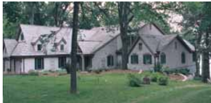
Below: Roman Electric installs and repairs electrical systems in a variety of new and remodeled homes.
