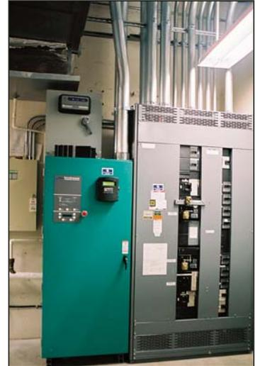
*Roman replaced ATC's main service switchgear and UPS transfer switch with minimal downtime.*
