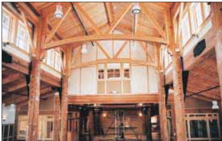
**The new Schlitz Audubon Nature Center features an impressive exhibition hall (left and right) with timber framing from trees harvested on-site.**
