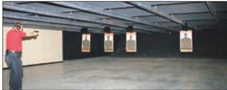
Sergeant Gregory Otto uses one of the three pistol firing ranges. The unique ventilation system completely exchanges the air every 87 seconds and provides a negative pressure so no air escapes from the room. The back wall contains several feet of shredded used tires to stop bullets.
